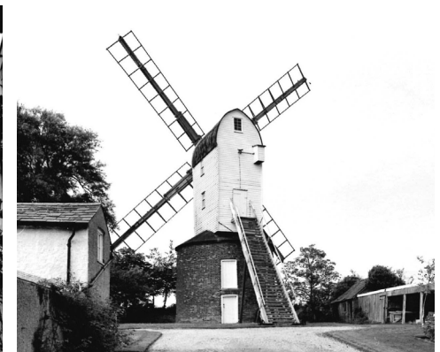
Figure 16 Ramsey Windmill in 1985, viewed from the south. Weatherboarding has been repaired and repainted, as have the stairs
